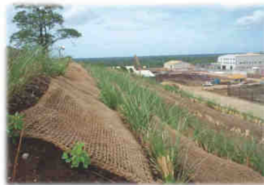
Photo 2: Strip sodding with hydroseeded areas covered in geofabrics (e.g. soil saver).
