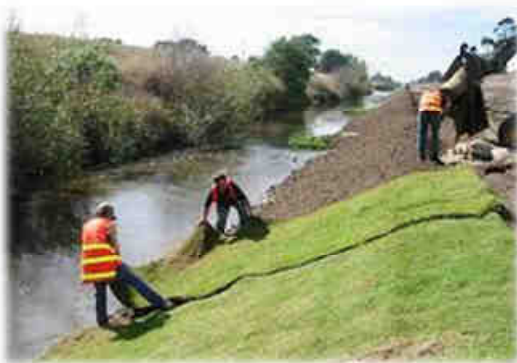
Photo 1: Layering of grass sods on a slope.
